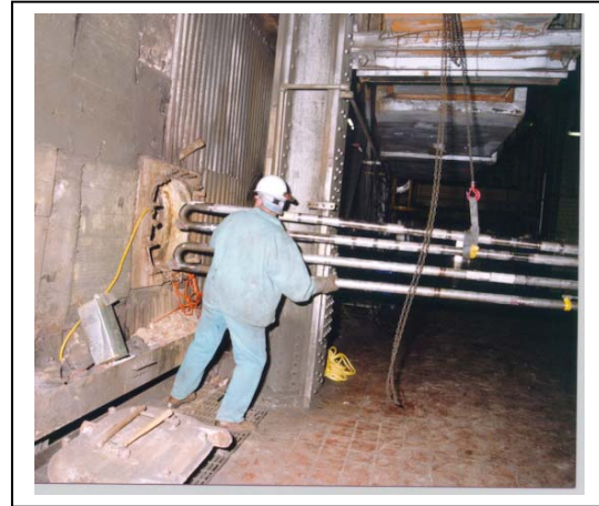
Figure 6: Installation into Niles Boiler
